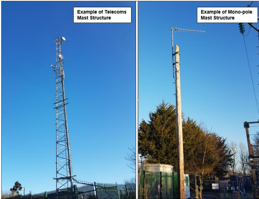
Figure 13. Example structures that could be used at a relay mast-site.
